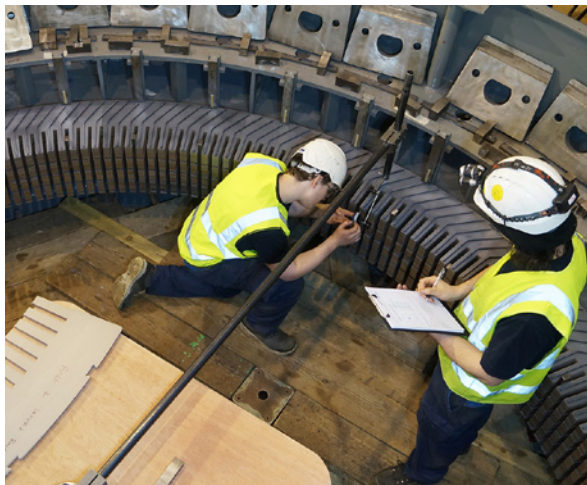
Sulzer rebuilt the core concentric to within 0.15 mm and circular from top to bottom to within 0.05 mm
